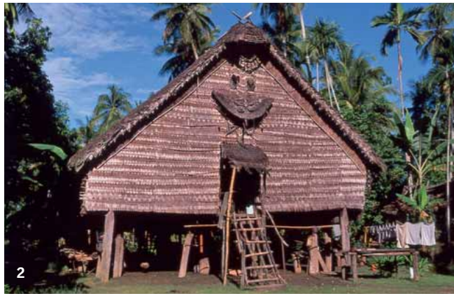
The Sago palm is the main building material of traditional Papua New Guinean dwellings. Posts are made from the trunk of the palm, wall shingles and the roof from the leaves, and floors from the skin of the trunk.
